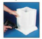
**7.** Secured caps in place. Drill two holes opposite each other, through cap and into column. Secure cap in place with screws.
