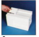
2. Locate top and bottom trim panels in recessed area of column quarter with grooves nearest ends of column section.
