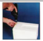
**4.** Drill a 1/8" hole through column and attach trim panel to the column with a No. 8 x 3/4" Lg. Phillips flat head stainless sheet metal screw furnished. Follow the same procedure on all four sections.
